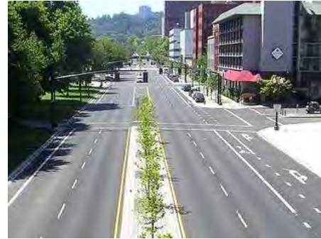
This street in Portland, Oregon previously had 4.0 m lanes, which were narrowed to accommodate bicycle lanes without removing a lane.
