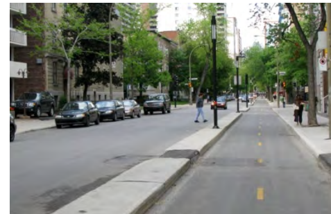
Cycle track with curb separation, Montreal QC.
