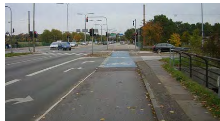
At this unsignalized right turn, the cycle track has dropped to a bicycle lane with blue coloration and pavement markings through the conflict area. A “Yield to Cyclists” Sign would further improve this intersection.
