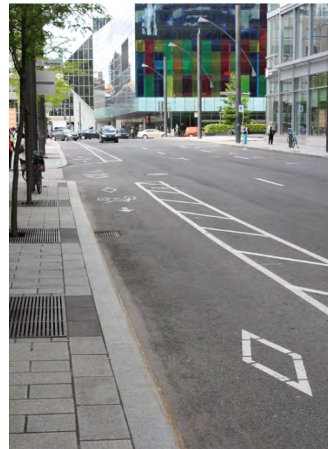
Montréal uses buffered bicycle lanes to protect cyclists from fast-moving traffic.
