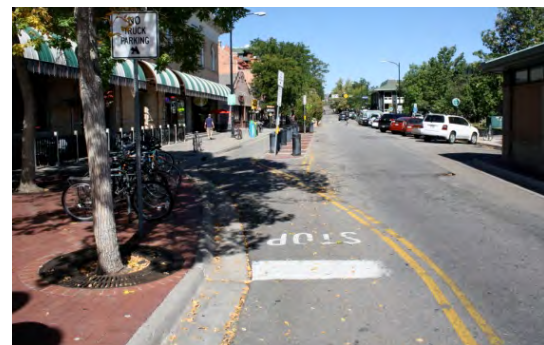
This contraflow bicycle lane in Denver, Colorado provides a key connection between bikeways.
