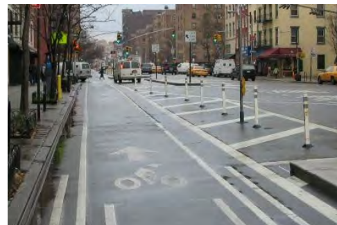
Cycle track with bollard separation, New York City.
