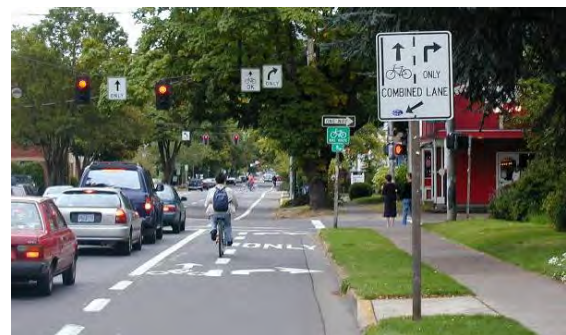
Shared bike-right turn lanes require warning signage as well as pavement markings to facilitate automobiles and cyclists sharing the lane.
