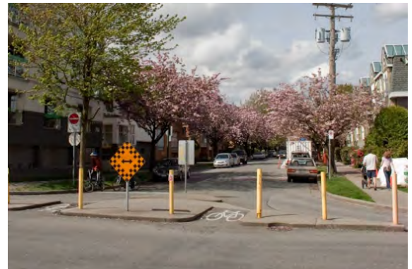
Right in/right out islands prohibit thru-vehicle traffic on a neighbourhood bikeway.
