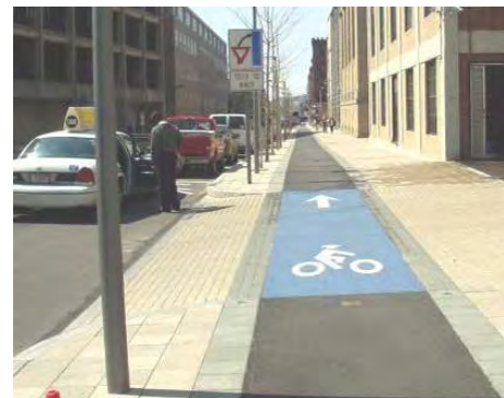
Coloured pavement informs bicyclists and drivers of a potential conflict area.
