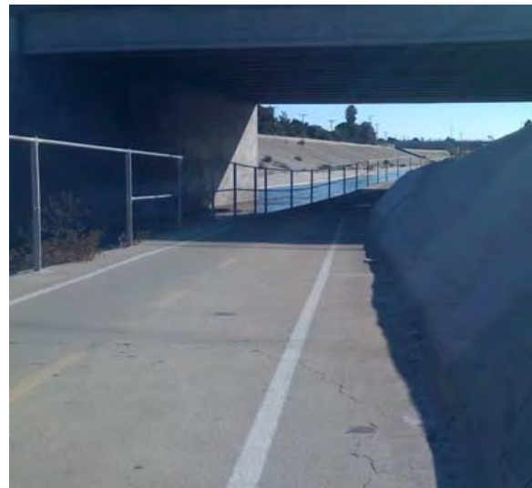
Undercrossings provide key connections and allow trail users to avoid a potentially dangerous at-grade crossing of a major street.
