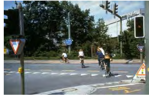
Left-turn from a cycle track on the right via bicycle-signal phase in Winterthur, Switzerland.
