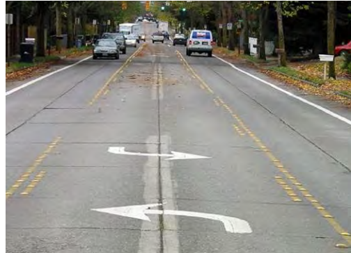
This road was re-striped to convert four vehicle travel lanes into three travel lanes with bicycle lanes.
