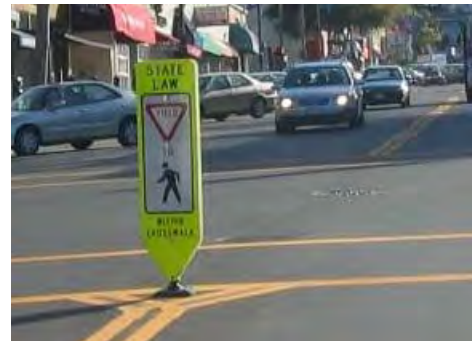
In-street yield to pedestrian signage.
