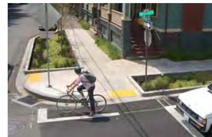
Bicycle forward stop bars encourage cyclists to wait where they are more visible.
