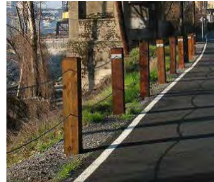
Post and wire fence.
