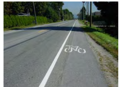
Shoulder bikeways can be indicated by pavement markings, and generally include signage.
