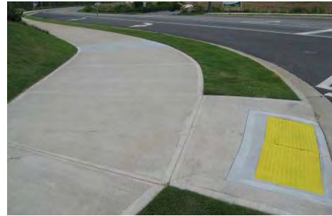
A diagonal curb ramp with detectible warning.
