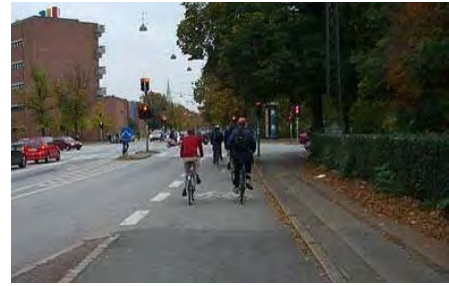
Cycle track dropping to bicycle lane before an intersection.
