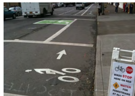
Bike box positions cyclists to make a left turn from a cycle track in Portland, OR.
