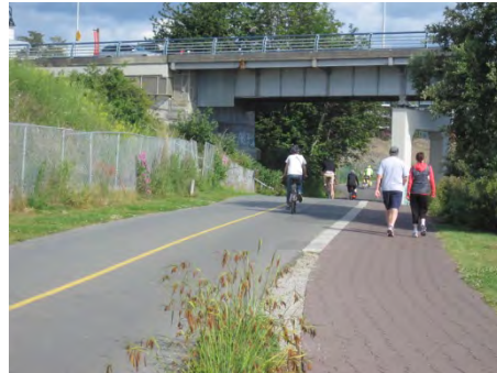
The Galloping Goose trail provides a separated pedestrian path and divided bicycle trail through high-use areas.
