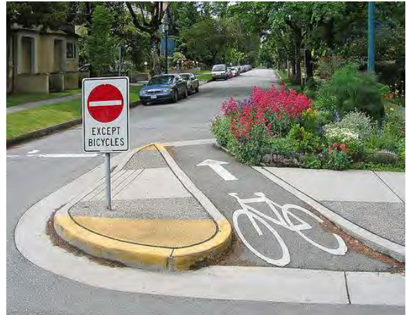
Choker entrances prevent vehicular traffic from turning from a main street onto a traffic-calmed neighbourhood bikeway.
