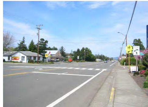
Advance stop bars alert motorists of pedestrians.
