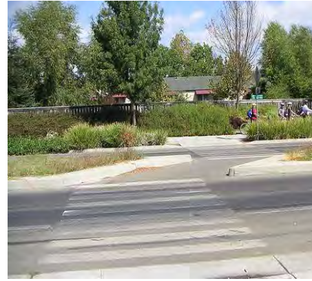
An offset crossing forces pedestrians to turn and face the traffic they are about to cross.
