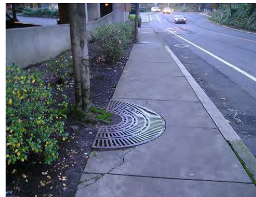
Tree well grates can create uneven sidewalk conditions.
