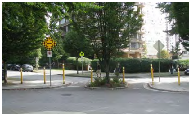
Traffic diverters prevent access to both directions of motor vehicle traffic.
