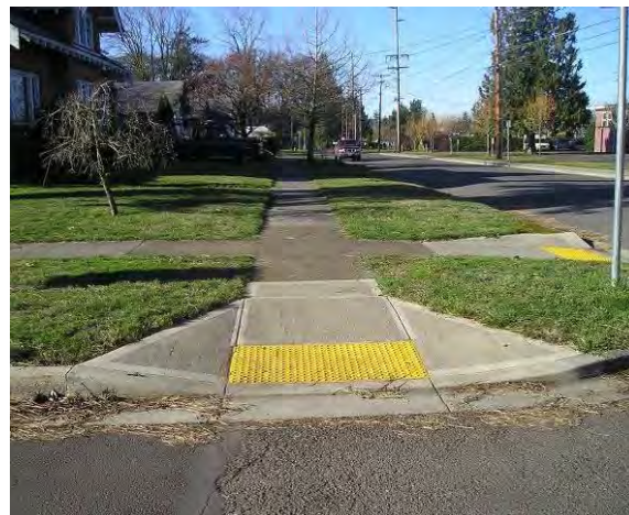
Example of an accessible perpendicular curb ramp.
