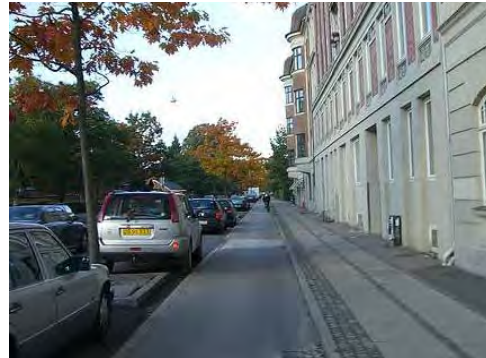
Cycle track with a parking buffer, Copenhagen.
