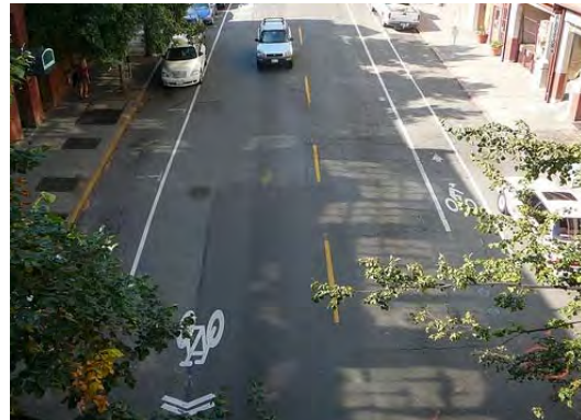
Cyclists traveling downhill can match automobile speeds and do not require additional separation, unlike cyclists riding uphill.
