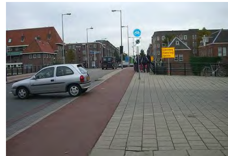
Cycle tracks should be continued through driveway crossings, improving visibility.
