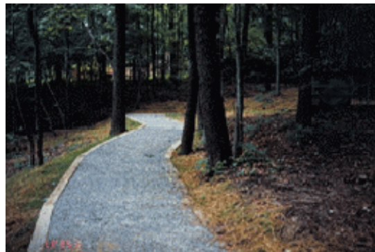
Crusher fines is similar to gravel and a common soft-surface trail material.
