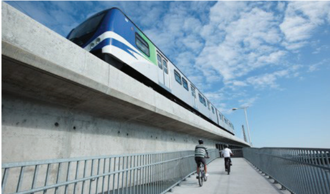
Canada Line Bridge, Richmond
