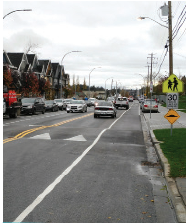
Painted bicycle lanes on 148 St between 64 and 72 Ave (Surrey)
