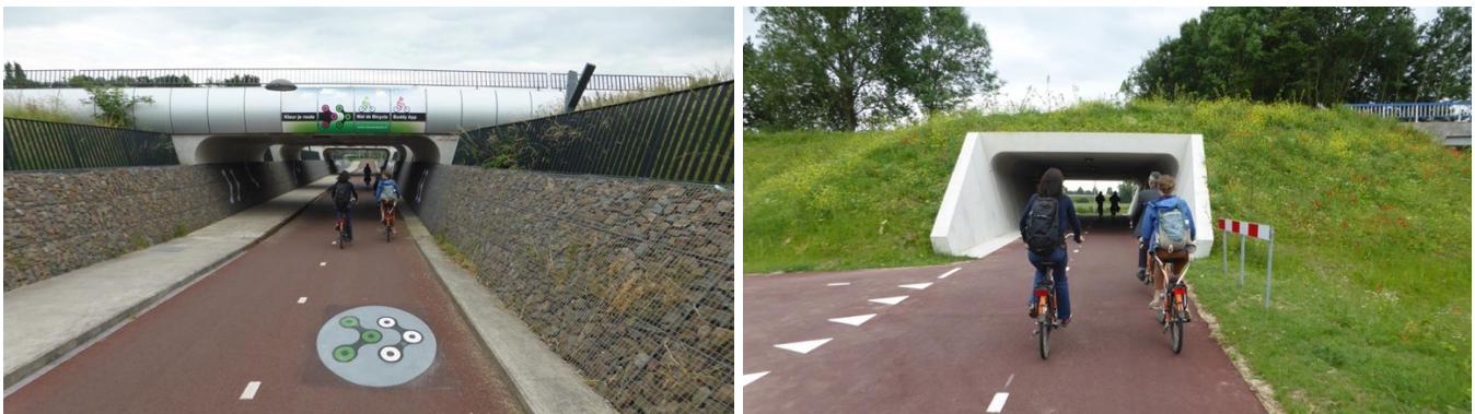
Figure 12: Tunnels along the Rijnwaalpad, the Netherlands: a tunnel under the A15 motorway, with outward leaning walls creating a feeling of roominess (left), and the Kattenleger tunnel, which makes the route 250m shorter and avoids crossing a busy road (right) 201
